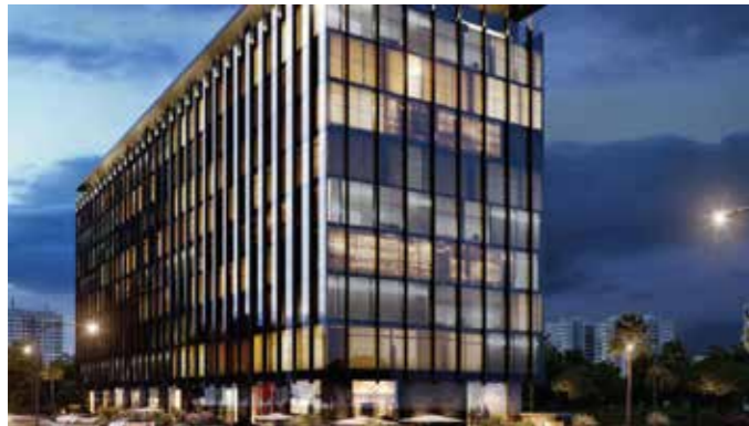
↑ Panchshil Balewadi Commercial, Pune
